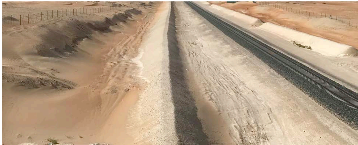
Figure 5. DB system protecting railway track in UAE.
