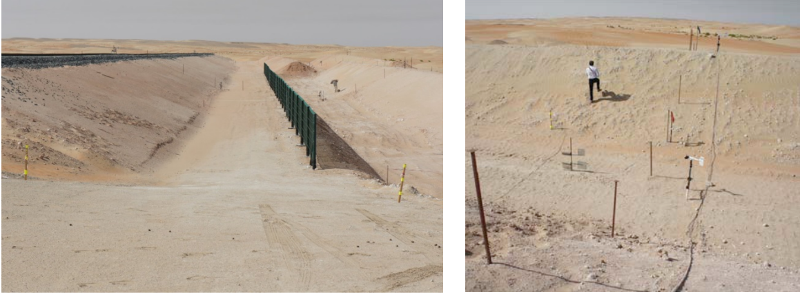
Figure 2. ER Stage 1 trial field view (left) and monitored cross section (right).
